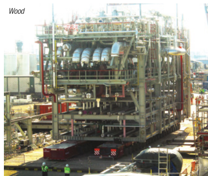
FIGURE 1. It is not the size of the project that makes it a good fit for modular construction, rather it often has to do with the complexity of the project. Shown here is a complex module designed and built by Wood
